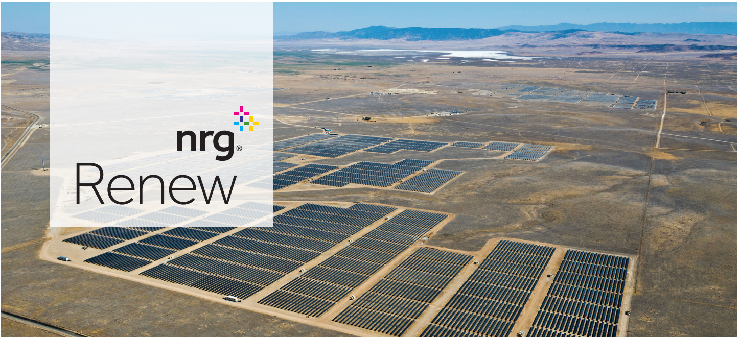
California Valley Solar Ranch Project
